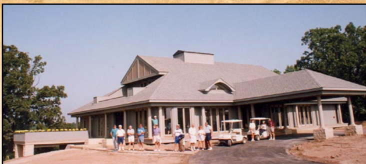
The clubhouse and Hanneken's Restaurant under construction.
