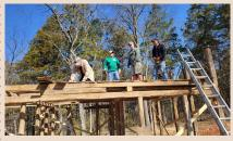
The progress report from this week shows additional decking being installed in the loft of the barn. The back half of the structure is almost complete and outside posts for the front half of the barn are now being put into place. After the front section is completed, the next major step will be the placement of the barn's roof rafters.
