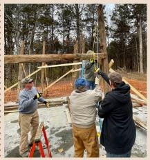
With more cooperation from Mother Nature, the barn crew was able to mark a special milestone event this week. The first crossbeam (the one which will support the loft) was put into place. The picture above shows the new beam being hoisted into position. The mortise and tenon joints from the 19th century went together just like they did when the barn was first built.
